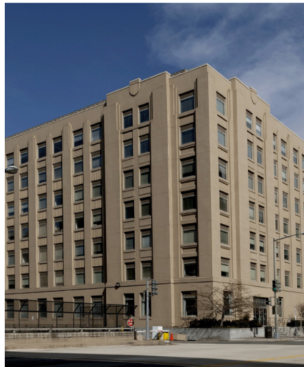
301 7TH STREET SW GSA Regional Office Building Date Listed: 4/10/2025 Status: SOLD Square Feet: 940,000
