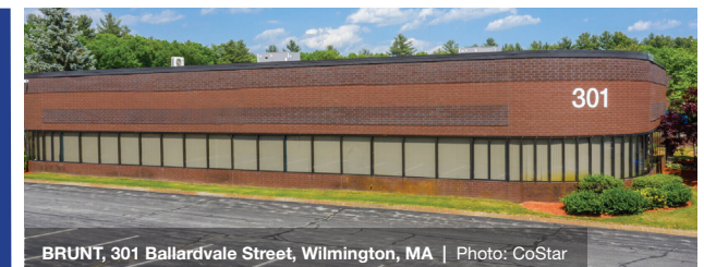
BRUNT, 301 Ballardvale Street, Wilmington, MA | Photo: CoStar
