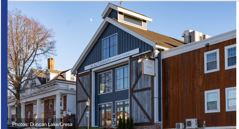
Photos: Duncan Lake/Cresa
