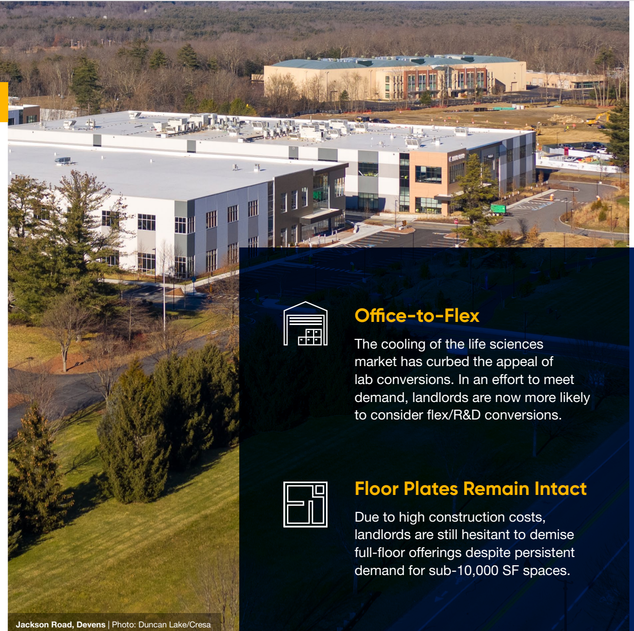
Jackson Road, Devens | Photo: Duncan Lake/Cresa
