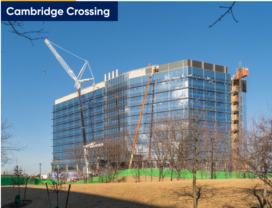
Cambridge Crossing Construction | Photo Source: Cresa/Duncan Lake
